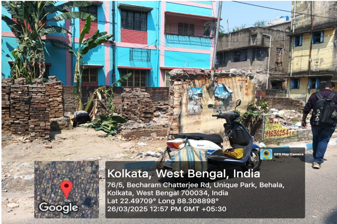
Construction work in progress
