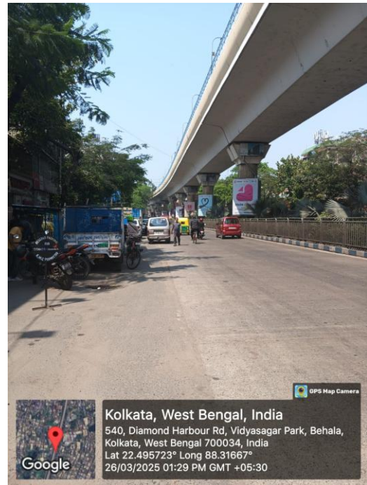
Main Communication (Diamond Harbour Road)
